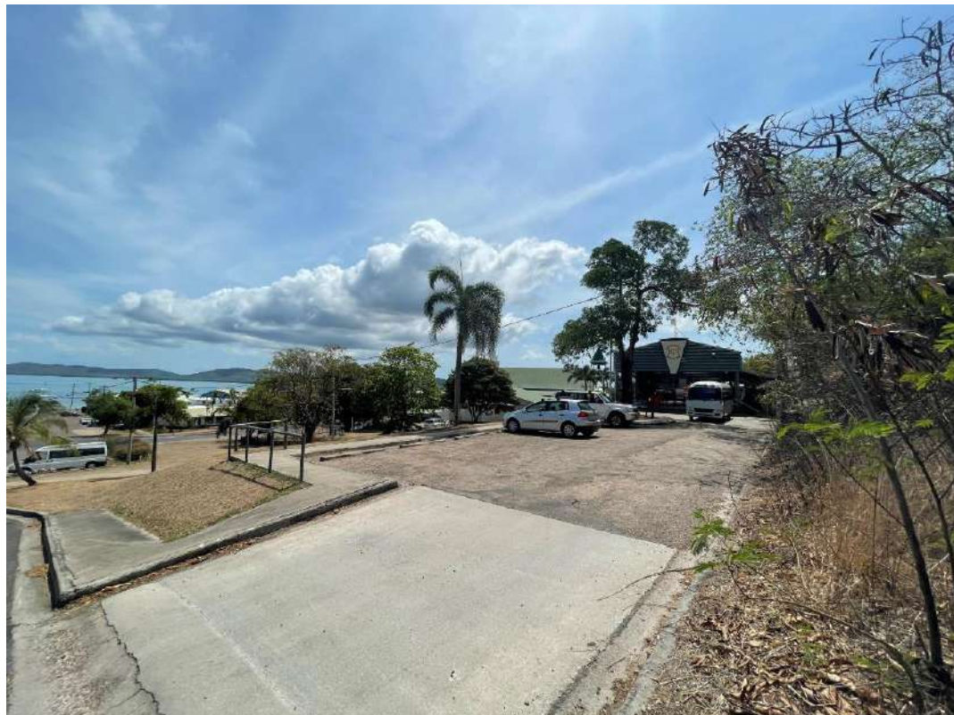
Figure 22: View D from Normanby Street and school driveway (AHS, 2020).
