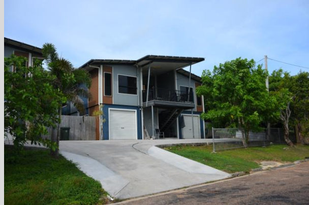
✓ 6.1 This building includes windows and a balcony in an elevated position.
