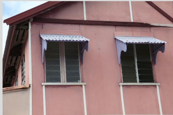
✓ 2.1 Window hoods providing sun protection to windows.
