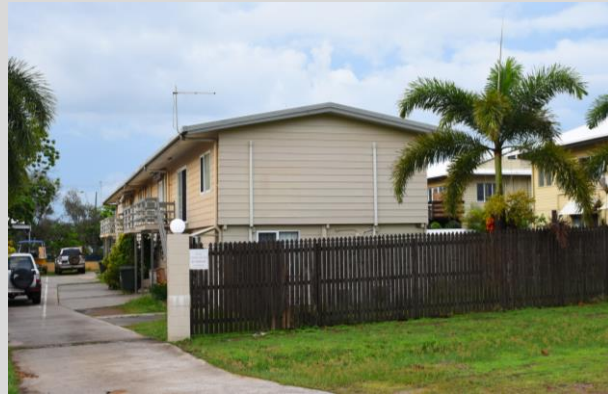
✗ 6.2 This building includes a large blank wall, small windows and limited outdoor areas.
