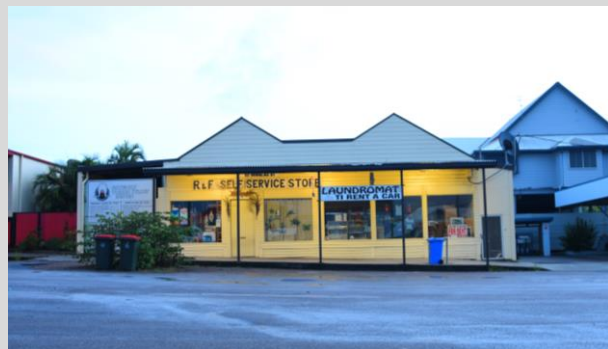
✓ 11.3 Lighting and signage used to assist in navigation and visibility.
