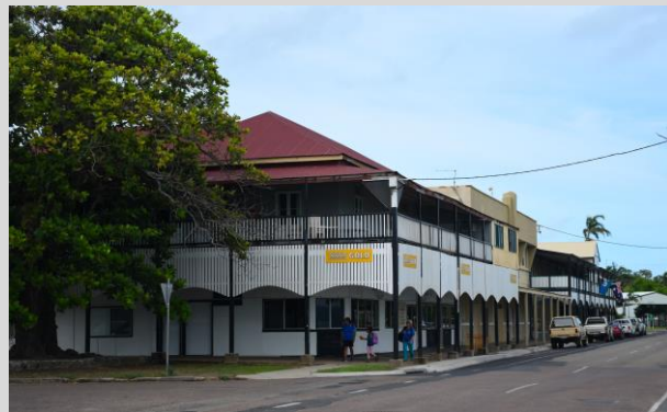
✓ 3.2 Consistent awnings along a street promote pedestrian activity due to weather protection.
