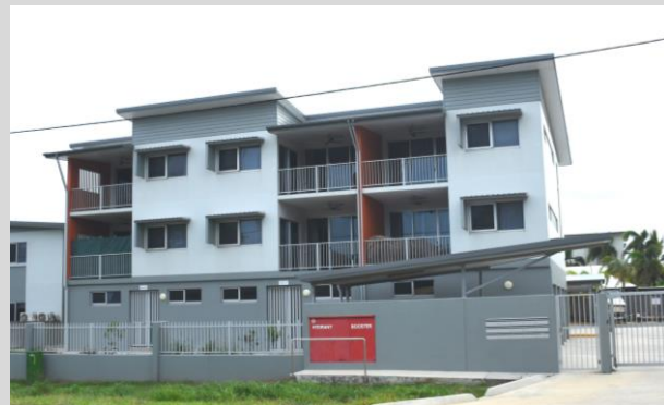
✓ 2.2 Window hoods and recessed windows through the use of balconies provide shading.
