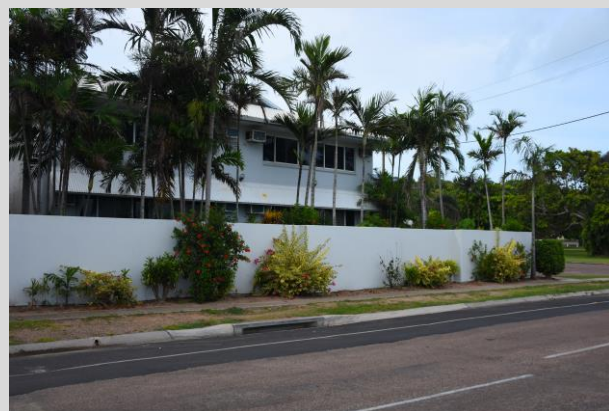
✗ 10.3 A large blank wall to the street prevents casual surveillance
