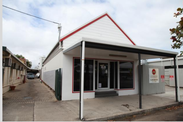
✓ 9.1 The driveway in the left of this photograph promotes visibility of activities along the side and rear of the site .
