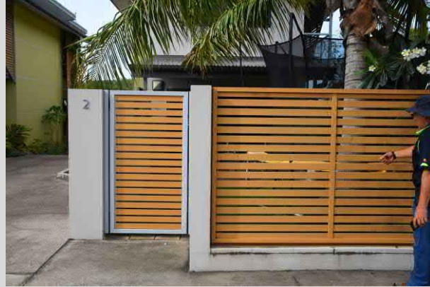
✓ 10.1 Fencing is used to provide boundary delineation whilst maintaining surveillance due to its transparent design.
