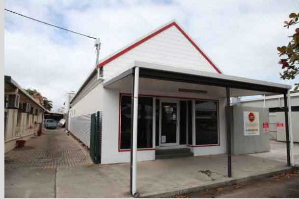
✓ 9.1 The driveway in the left of this photograph promotes visibility of activities along the side and rear of the site .
