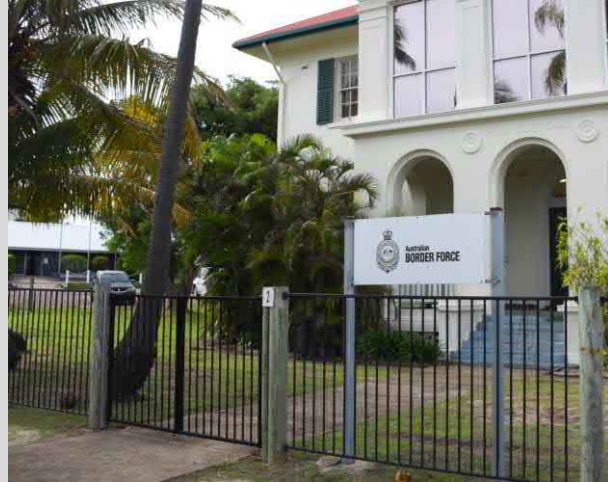
✓ 11.1 Signage (name and number) is used to identify premises.
