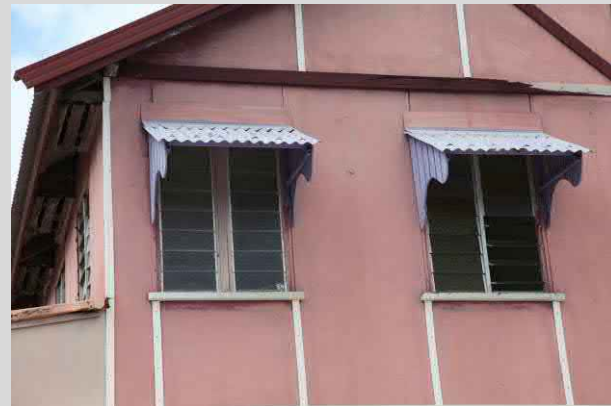
✓ 2.1 Window hoods providing sun protection to windows.
