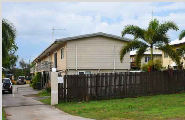
✗ 6.2 This building includes a large blank wall, small windows and limited outdoor areas.
